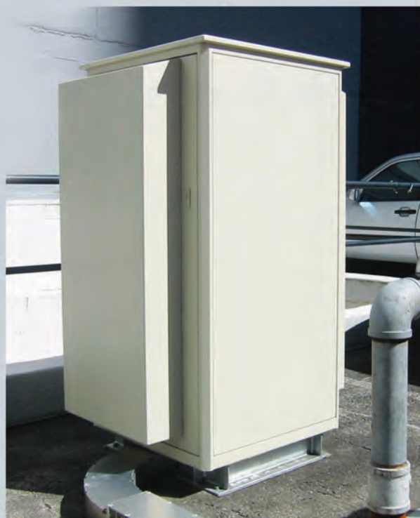
ALCATEL LUCENT REPEATER SITE using forced filter cooling with additional silencers provide < 45 db
