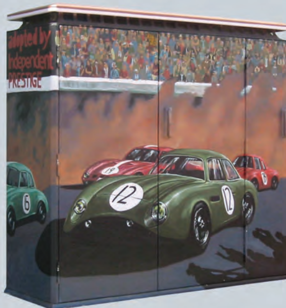
NOKIA 480 LINE SDH with integrated 1100W heat exchanger. Now painted to deter the graffiti artist.
